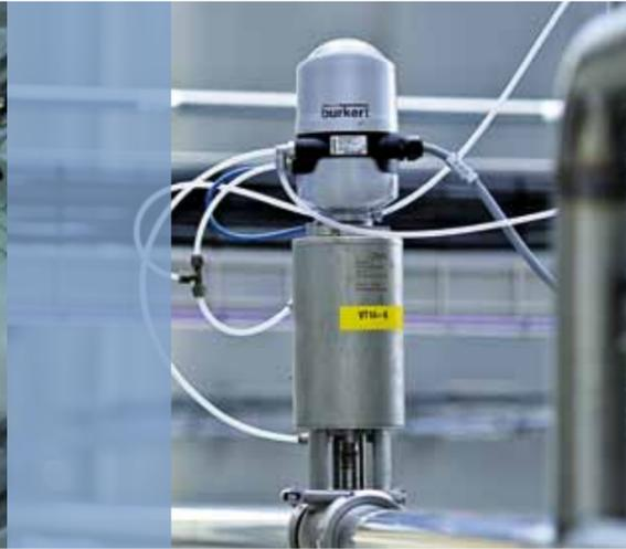
Flow management is ensured by agrifoodstuff valves, controlled by fieldbus
