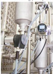
Caption 2: FLOWave enables continuous monitoring of the cleaning procedure, which makes it a valuable quality assurance tool.
