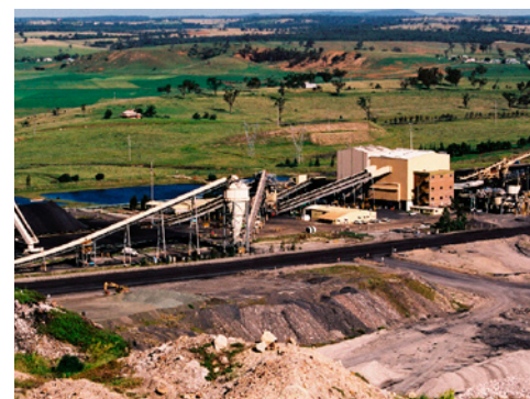
Mt Thorley Warkworth coal handling and preparation plant.
