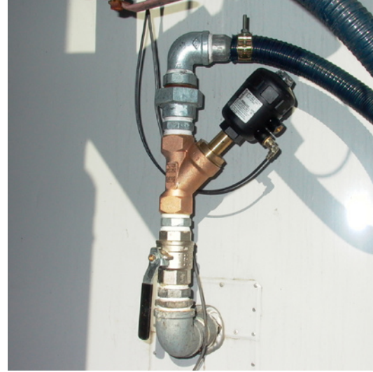
A simple glycol flow system, with Type 2000 process valve and two isolating valves at the tank. Controlled via temperature controllers on each tank and connected to pneumatic control panels.
